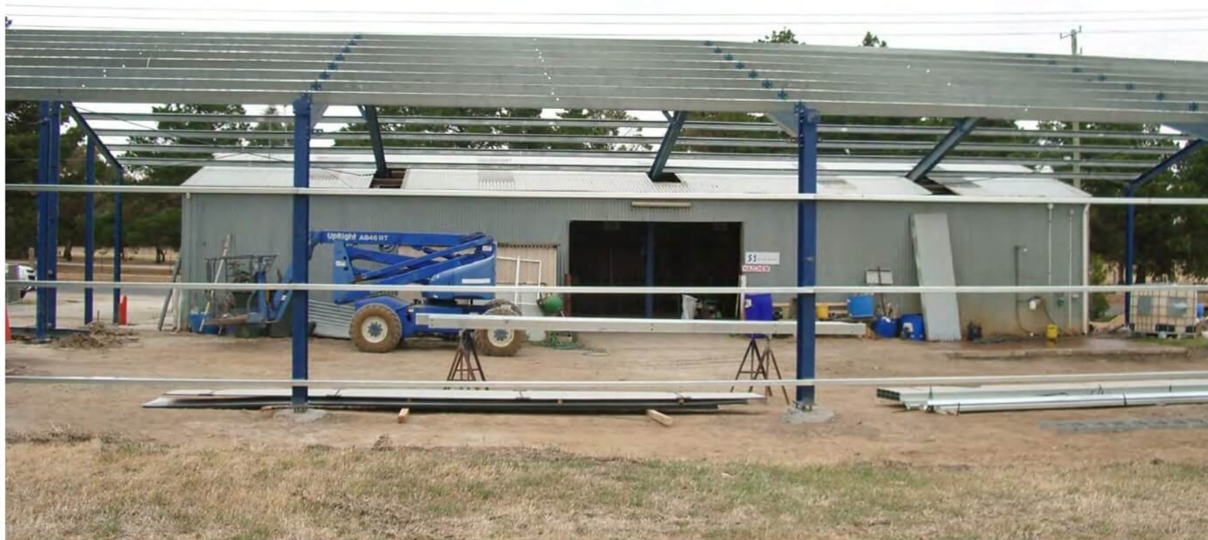
Early stage in the construction of the greenkeeper's shed
