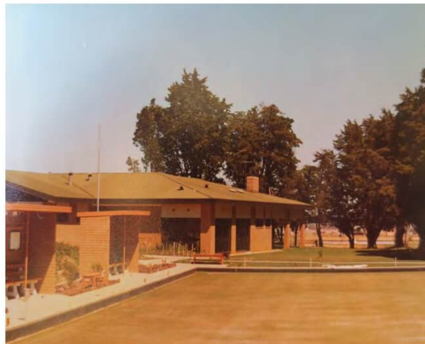
Photo above before function room added to the clubhouse Photos left and above taken from approximately the same position
