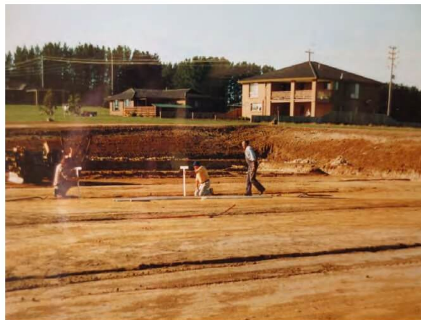
Construction of the new green in progress
