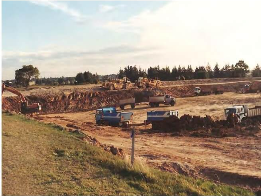
Excavation of the dam adjacent to the ninth fairway
